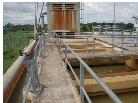
Iron removal process by aeration and filtration
