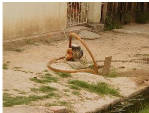
Water meters were replaced with pump!
