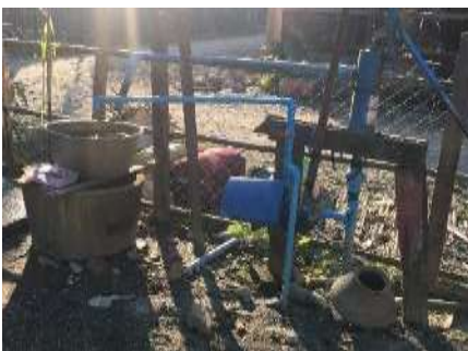
A tube well and pump at the front yard
