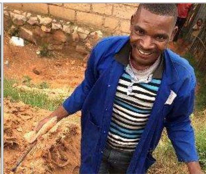
Staff with a hot iron bar for drilling on distribution pipe
