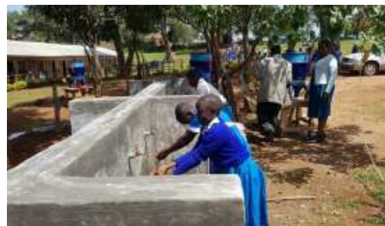
Construction of Water supply facility in a school (Kenya)
