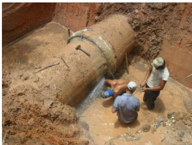
Figure 4 Repairing Leakage on transmission pipe
