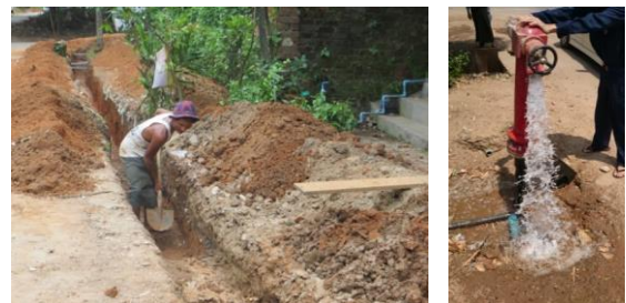
Figure 7 Digging for laying pipes & water supply after completion of the project
