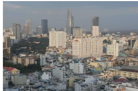
Skyscrapers are constructed in Ho Chi Minh City
