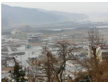
Destroyed central area by Tsunami
