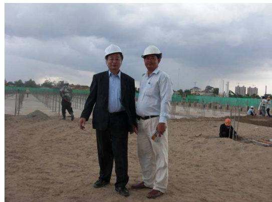
Construction field of new water treatment plant In Phnom Penh
