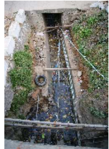
Right: Messy installation of distribution pipes, service pipes and electric lines. Stuck rubbish is one of causes of flood in rainy season.
