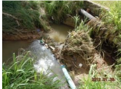
Photo 2: Bubbles on the water surface at crossing points of waterways
