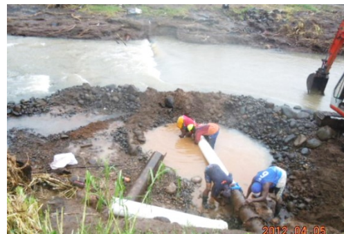
Photo 4: Piping work (repairing leakage) in water
