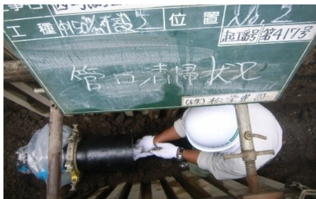
Picture-2 Cleaning inside pipe
