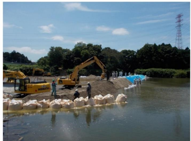
Construction work of the temporary soil dike in Kuji River
