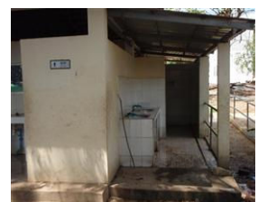
Toilet of hospital in rural Cambodia
