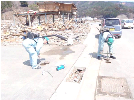
Checking valves by Staff of SWWB (Ishinomaki City)
