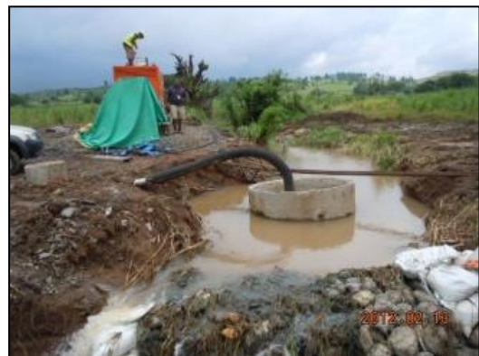
The emergency & temporary intake from the stream on the way to the raw water pipeline at Ba. (There is the generator in the left & upper part of the picture.)
